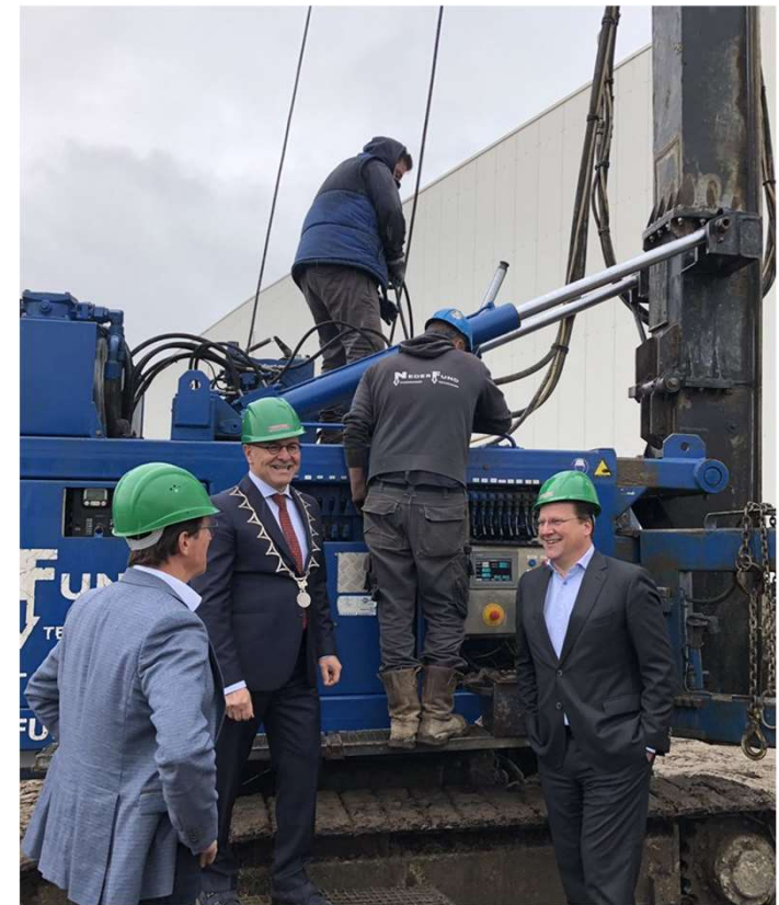
First pile of our new fresh produce distribution centre in Veghel
